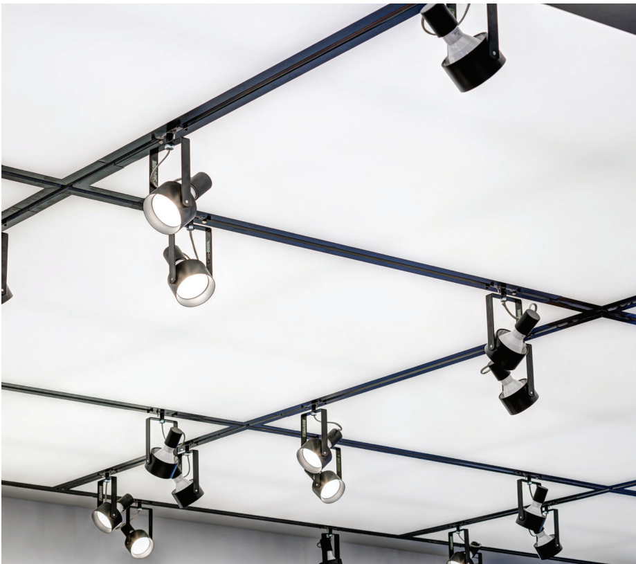
Track luminaires were added to provide the feel of a fashion runway
